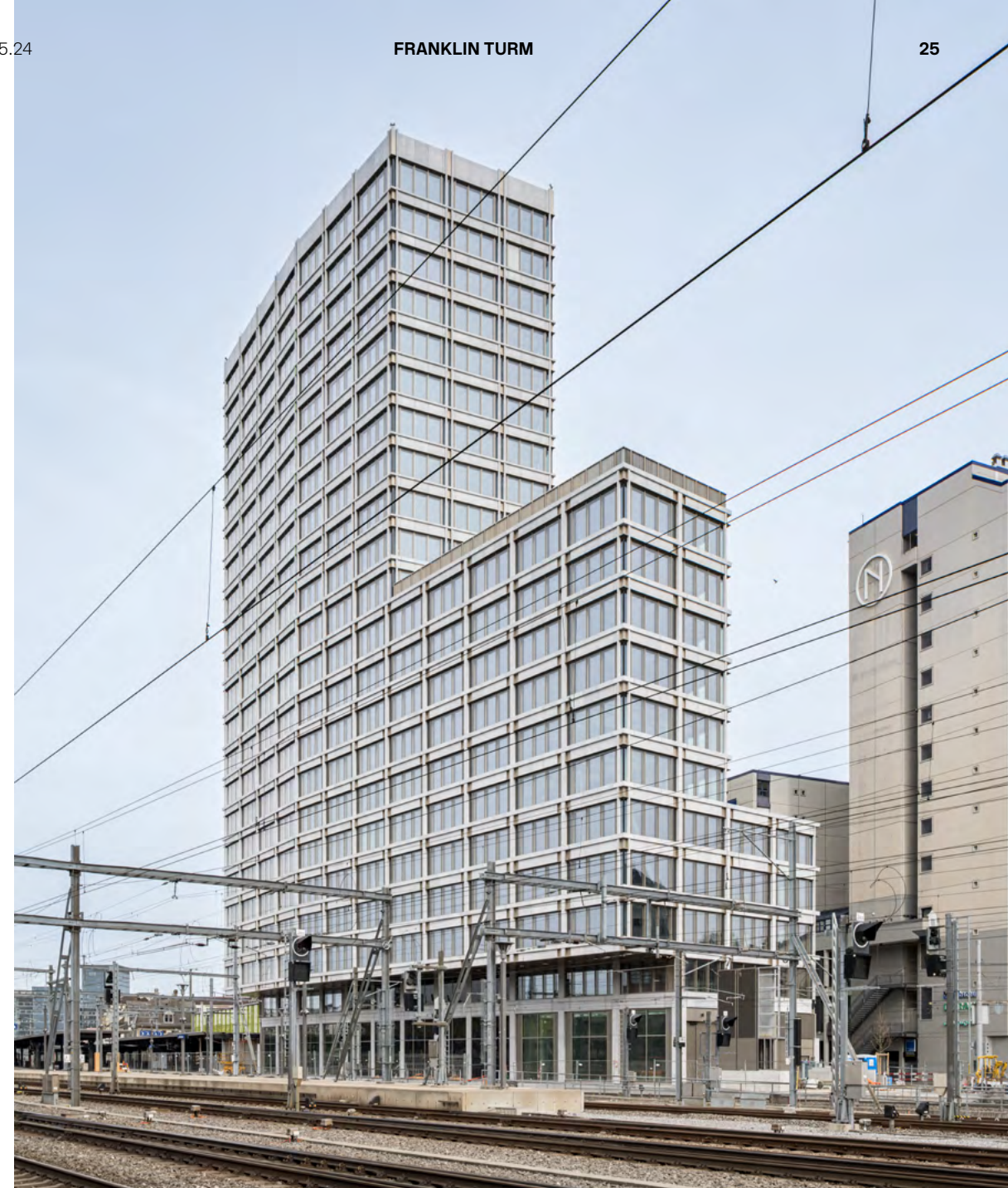
Staggering the heights along three levels softens the building's volume and connects the lofty with the low.
